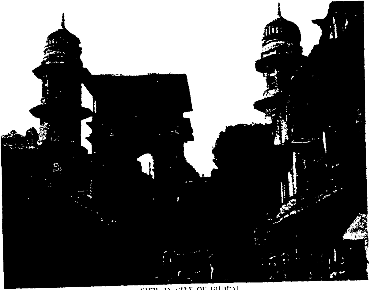
VIEW IN CITY OF BHOPAL
